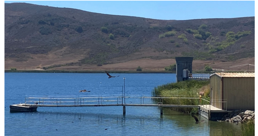
Existing Floating Maintenance Dock And Walkway
