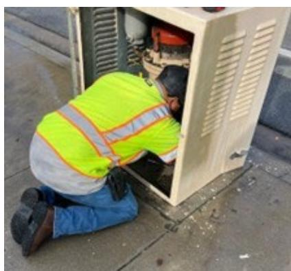
and Arneill Road in the City of Camarillo. Upon inspection, staff observed damage to the air and vacuum valve cabinet and the one-inch brass fittings on the air and vacuum valve, possibly caused by a vehicle, although this could not be confirmed. Staff successfully isolated the air and vacuum valve, completed the necessary repairs, restored the system to service, and replaced the damaged cabinet.
