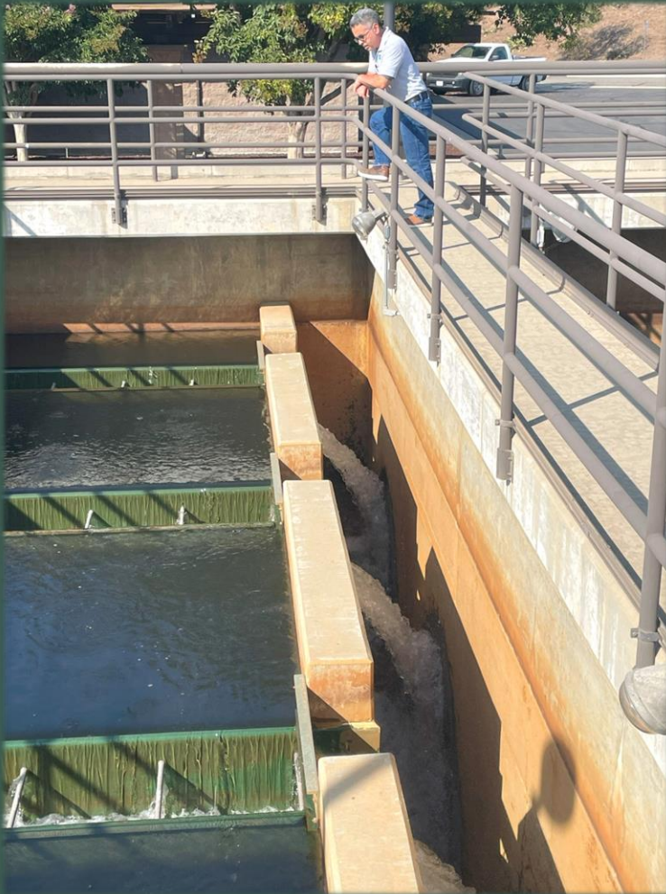
Rafael Medina overseeing a filter backwash
