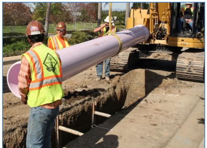
City of Oxnard Recycled Water Pipeline Installation
