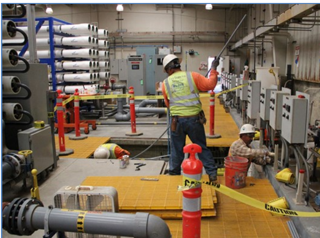
Construction at Port Hueneme Water Agency Groundwater Desalination Facility
