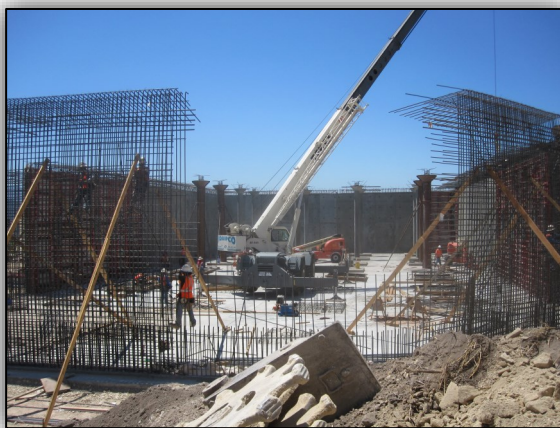
Thousand Oaks Reservoir
