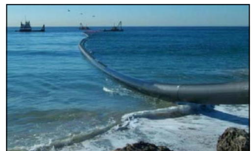
Ocean Outfall Construction
